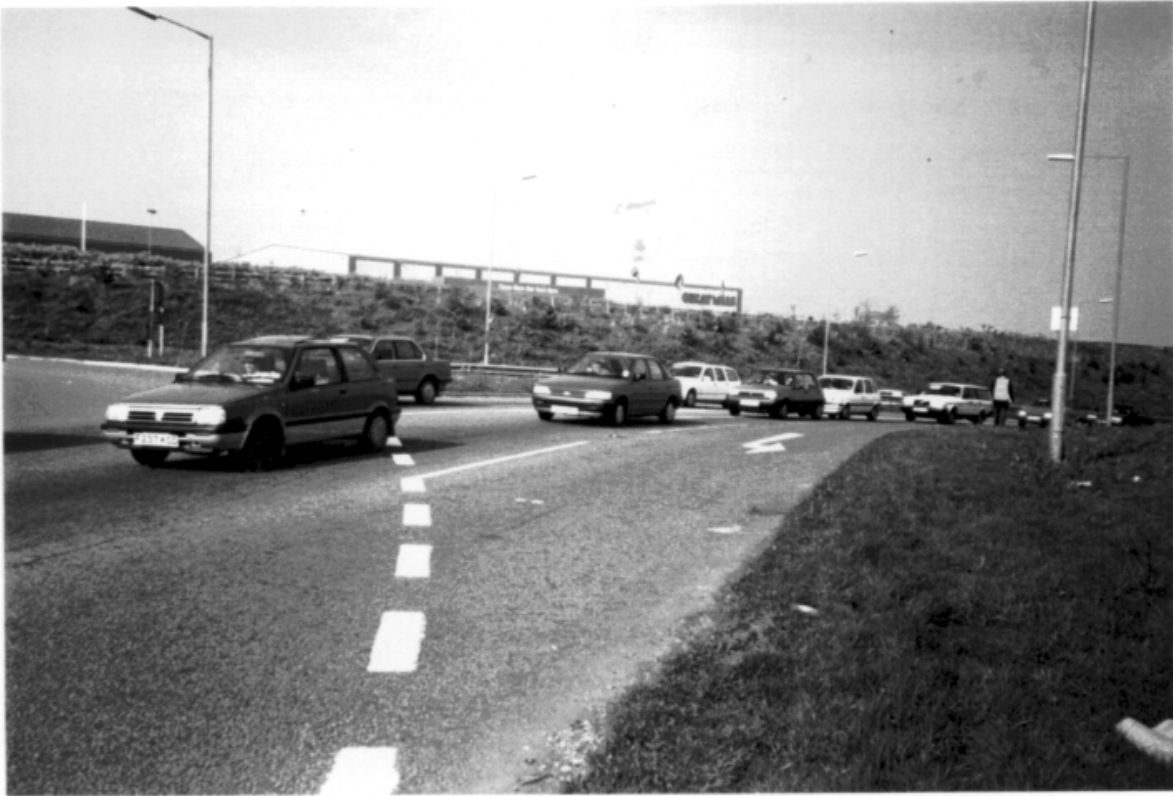
Photograph 1.1. Origin-Destination pattern of this pm peak traffic is such that the near-side flare section is virtually unused. ARCADY is 'blind' to this fact
