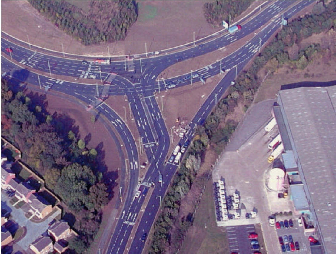
Photo of DRT junction – Swindon (Source Nuttall, 2002)
