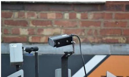
3.3 The detector was mounted on a primary 4m pole. We would normally mount the detector in the same position as a conventional MVD but there is an access point already installed on the signal head top bracket. We fitted a 4 in line top bracket where a far sided pedestrian head would be mounted. This gave us a good line of sight.
