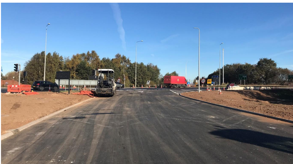
Figure 8 – Photograph of work nearing completion
